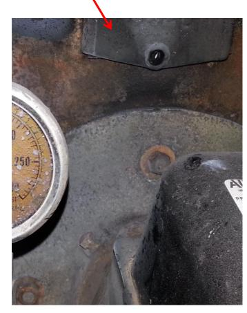
4) If oil pressure rises, but no ignition sound or combustion, issue is likely a like the transformer or a clogged nozzle - call SJ Fuel 718-855-6060.
